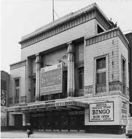
Plate 214 The Carlton Cinema, Essex Road, Islington, London, by George Coles, 1929–30. The façade is clad in cream faïence with vermilion, green, blue, and yellow embellishments. It has come down in the world. Photograph of 1973 (GLPL No. 73/2542).
